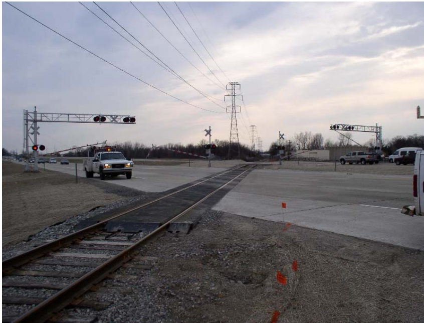
Highway Grade Crossing
